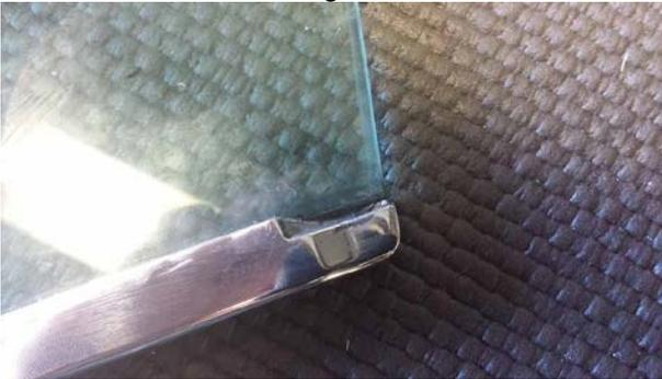
**13** Use black RTV to fill ends of channel wipe off excess as shown
